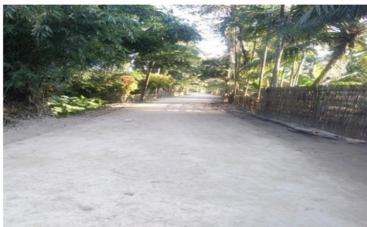
Figure - 5.5 Road of Nam Deuri village
