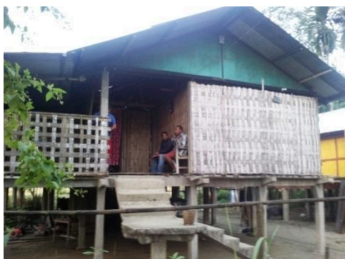
Figure: 3.2 A: The Chang Ghar of a Poor(APL) family
