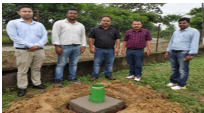
Figure 6.24. Installation of Ordinary Rain gauge at KVK, Jorhat, Assam
