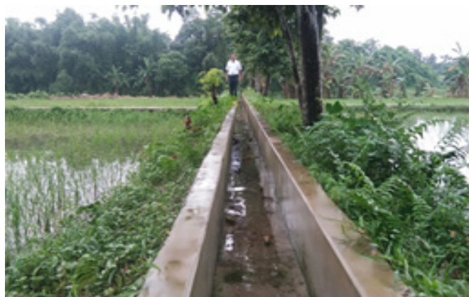
Figure 7.3. Construction of Irrigation canal under ICAR, AICRP Maize in RARS, Gossaigaon
