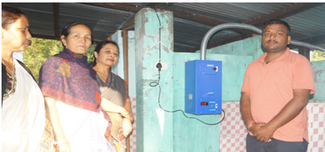
Figure 6.39. Installation of incinerators at a girls' school
