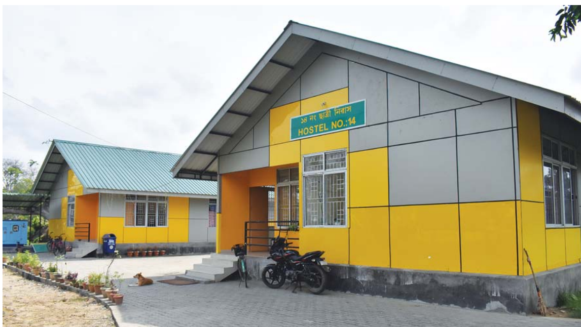
Figure 7.1. The new Girls Hostel (Hostel Number 14) in Jorhat
