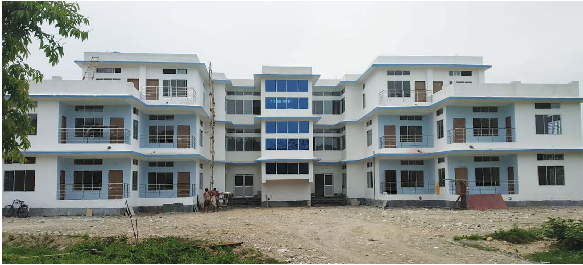
Figure 7.8. Construction of 3 Storied Staff Quarter at LCVSC, Joyhing
