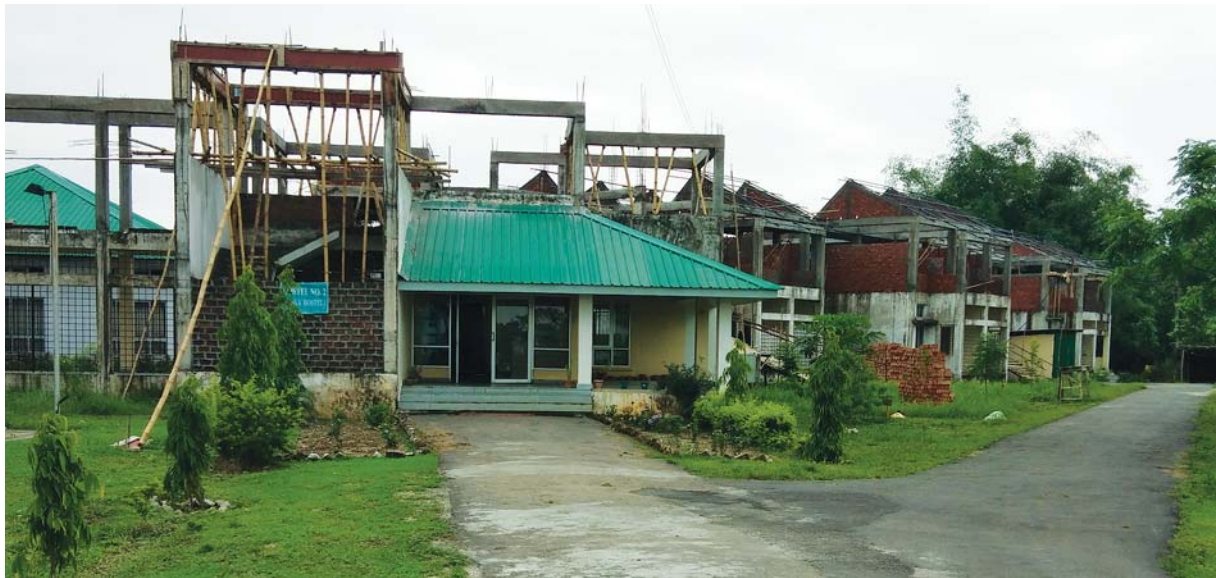
Figure 7.4. Ongoing construction work of Girls Hostel at SCS College of Agriculture
