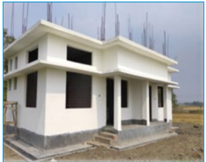
Figure 7.3. Employee's Quaters under construction, CH
