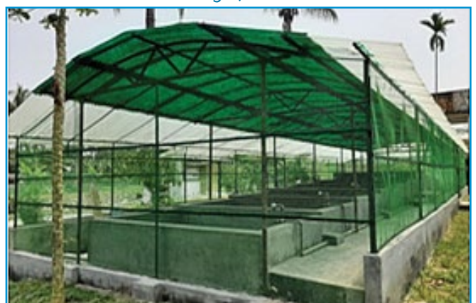
Figure 7.6. View of the innovative design of hatchery for Anabas developed at FRC, Jorhat, under TSP
